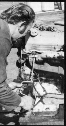
2. Next, the inlet and exhaust manifolds are removed. A socket set is essential for this job as the securing bolts are deep within the castings. The inlet manifold is retained for use on the marine engine, the exhaust manifold joins the scrap pile.
