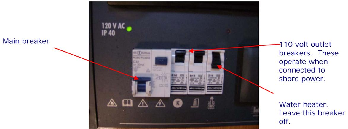
Island Beat is equipped with 2 110v outlets, one located by the 12 volt and 110 volt panel and one located in the galley. These will operate when the boat is connected to shore power or when you use the inverter. See next page for further details.
